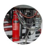
Cylinder mounting location and extinguishant selection is installation dependent.
